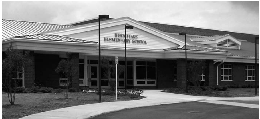
The LEED Green Building Rating System was used as a design guide for the Hermitage Elementary School in Virginia Beach.
